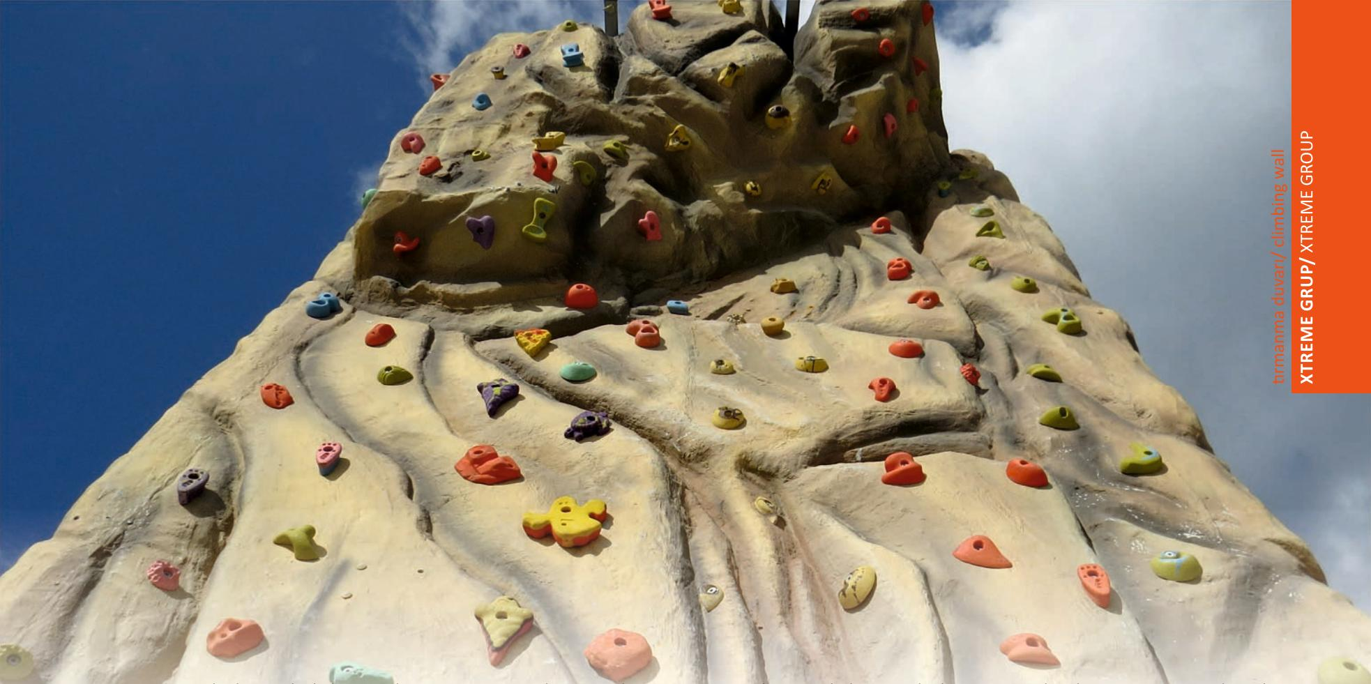
Sport climbing which has modern, innovator and active identity is accepted as sport of the new century in the World. Climbing wall is formed by holds placed on polyester or plywood panels and this polyester panels or plywood panels are build on steel constructions. For each level of user many routes in different difficulty levels on these walls can be created by adjusting number or dimension in-between holds and changing aim of the wall.
